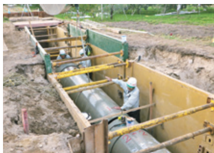
FRPM 管布設状況①
